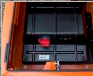
Battery cut-off switch
